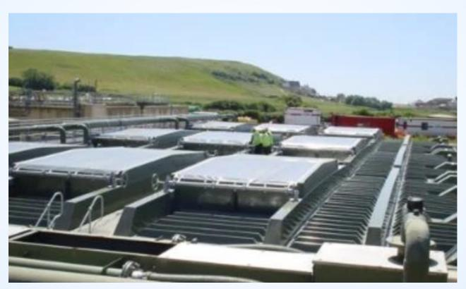
The operation of the fabric section is designed to be a one-person procedure and to require minimal effort. With only 3 moving parts, maintenance is kept to a minimum.
